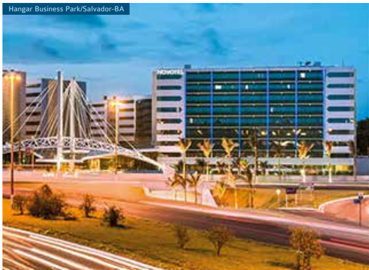
Hangar Business Park/Salvador-BA
